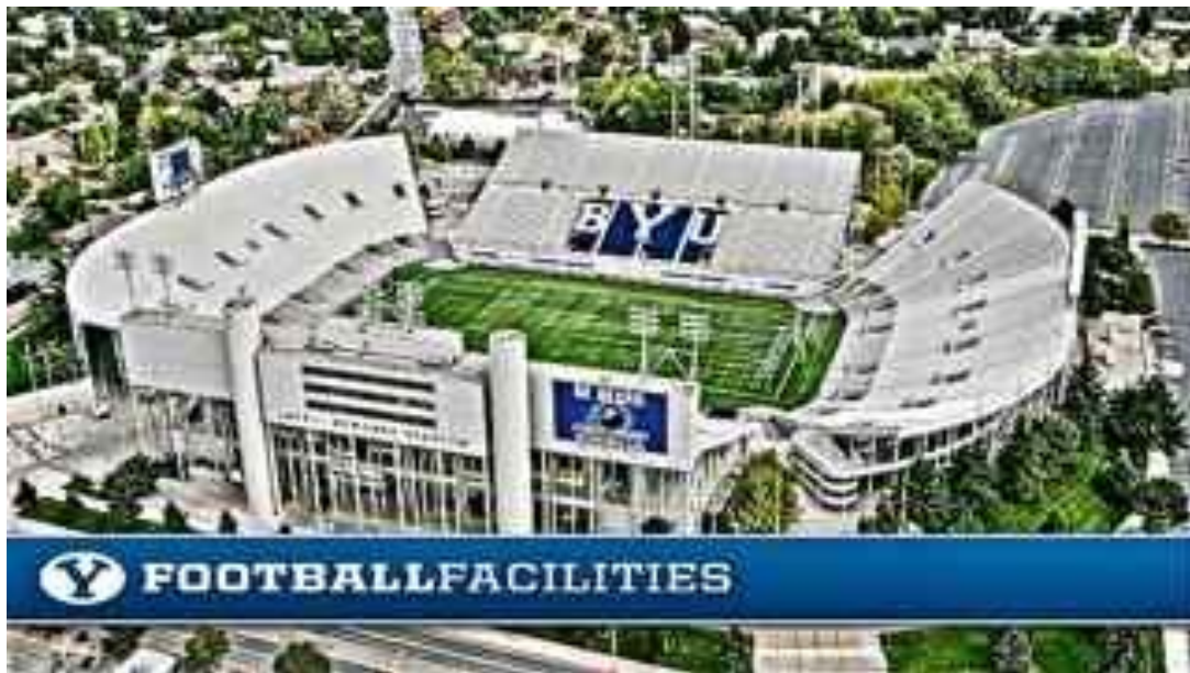
LAVELL EDWARDS FOOTBALL STADIUM SEATS 64,470 http://byucougars.com/facilities/football
